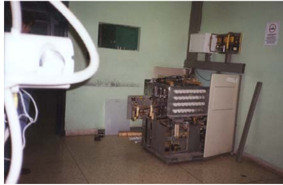
Vanlig syn: Under reparation.
