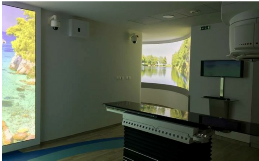
Fig. 3: Linear accelerator installation (courtesy Stavros Niarchos Foundation)
